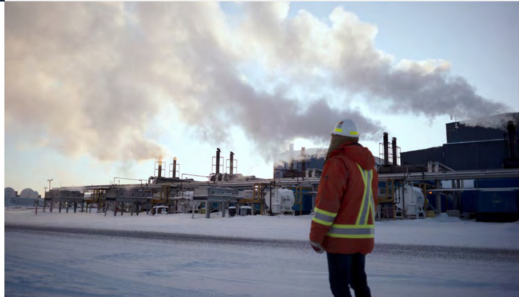
Employee looking onto the exterior of the Heat Recovery Unit, Gahcho Kué Mine, Canada. The waste heat generated from powering the processing plant is captured and recycled to heat the rest of the camp.
