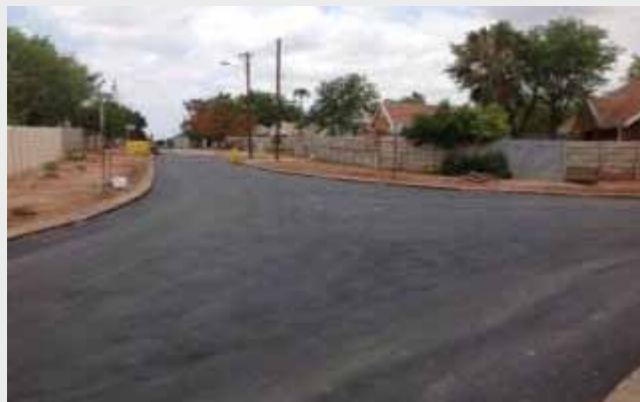
↑ VENETIA MINE UPGRADED A NUMBER OF INTERSECTIONS IN MUSINA.
