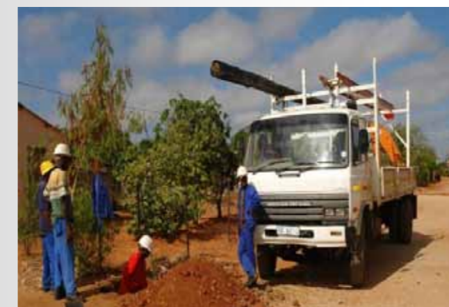
WORKERS PLANTING POLES FOR THE ELECTRIFICATION PROJECT IN MUSINA.
