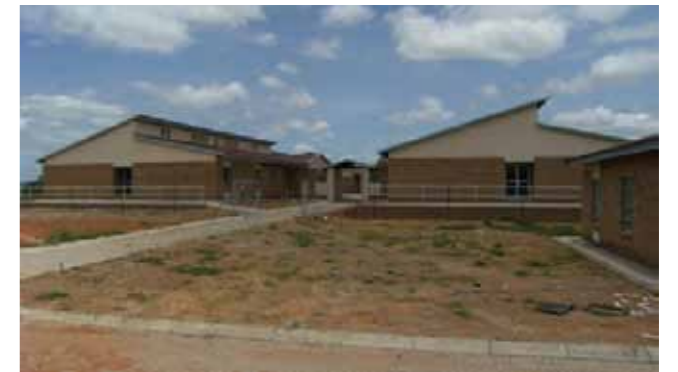
↑ RATANANG SPECIAL SCHOOL, UPGRADED BY VENETIA MINE.
